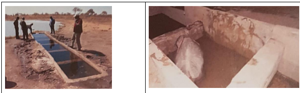
Figure 10-1: Existing troughs and their pitfalls
