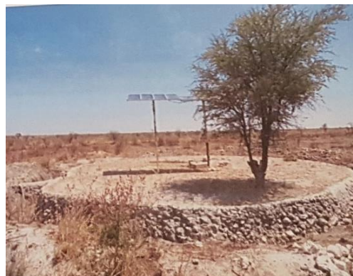
Figure 10-2: Inappropriate earlier water point design and appropriate elephant proof water point
